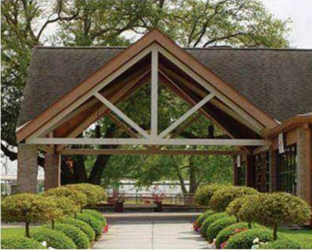
Trusses are commonly used to support roofs.
